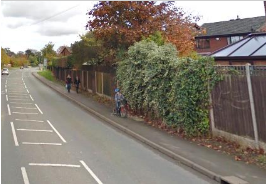
Figure 2-12: Narrow footways on A458 Welshpool Road (Source: Google Maps Street View)
