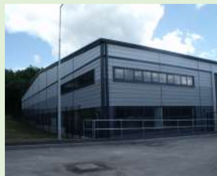
T54 – Plot 5c TWC industrial unit – Operational – Filtermist
