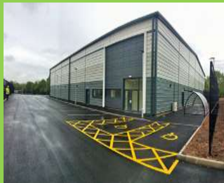
T54 – Plot 5a TWC industrial unit – Operational
